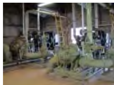
Pump for fire extinguishing (driven by engine when power failure happens) (Niigata Plant)
